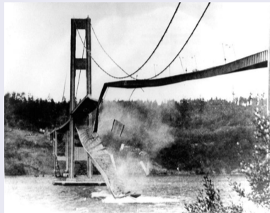
Figure 1: Resonant vibration of Tahoma Narrows Bridge
